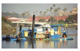
DEL MAR — Restoration of the San Dieguito Wetlands is now in the final phase of construction. The five-month project, which began Feb. 15, will dredge approximately 85,000 cubic yards of sand currently clogging the San Dieguito River channel, resulting in a better exchange of water from the ocean to the new nature preserve.
