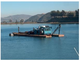
During August, the public can expect to see a floating dredge placed into the inlet channel. This specialized dredge is ideal for the San Dieguito Restoration Project because it is small, operates with minimum emissions and makes very little noise in comparison to other dredge equipment available. The dredge will first operate east of the Jimmy Durante Bridge and will pump the sand to a stockpile area where it will be dried and placed on upland sites that will be planted with
